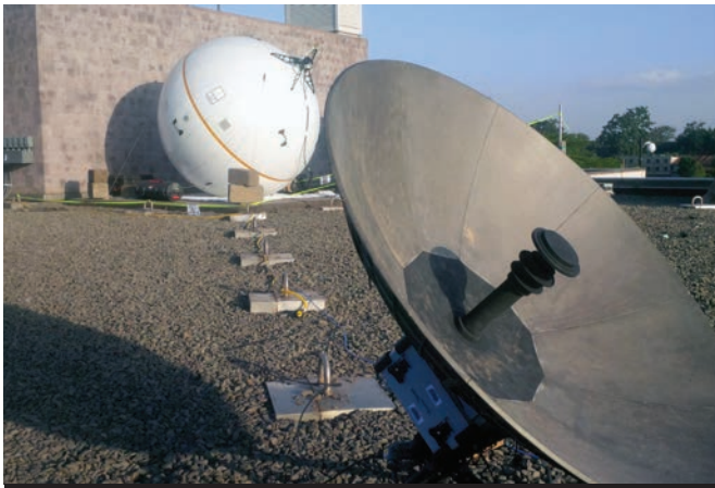
A U.S. Marine (far right) watches as DS security engineering officers oversee the set up of this Fly-Away, Very Small Aperture Terminal (in foreground) atop a U.S. Embassy in Africa. (U.S. Department of State photo)
